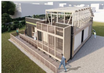
The HDU design consists of three major components: Living rooms, the Wintergarden and the Rooftop. It is built on a small plateau to represent the connection from the residential building to the vertical extension and includes the second story of the extension, including the Rooftop.
