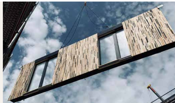
Façade element with preinstalled cladding and windows by the Team from Stuttgart. © coLLab / SDE 21/22
