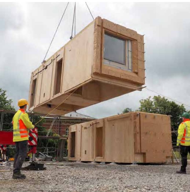
Module assembly by the team from Aachen: The second of six room modules in total is assembled. © LOCAL+ / SDE 21/22
