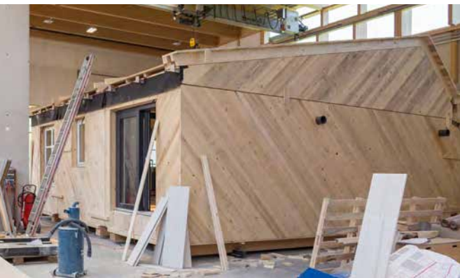
Diagonal formwork made of solid wooden boards by the team from Karlsruhe.
