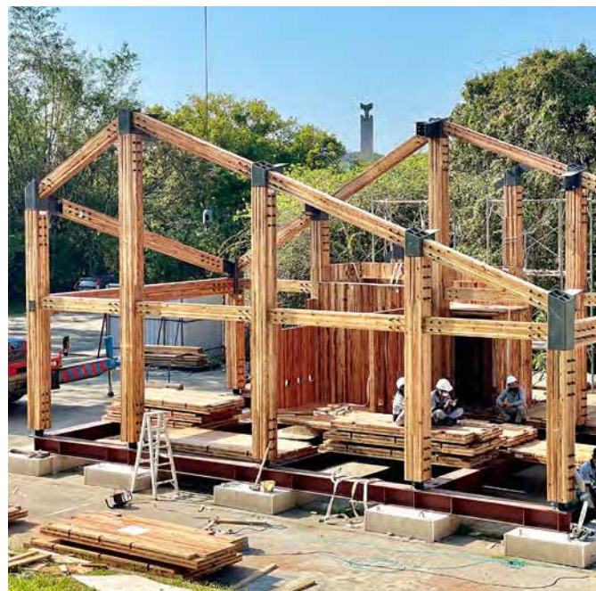
Timber frame made of cedar as the primary load-bearing structure. The Taipei team used small-scale elements.
