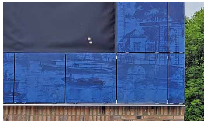
Curtain walls with coloured PV modules:
